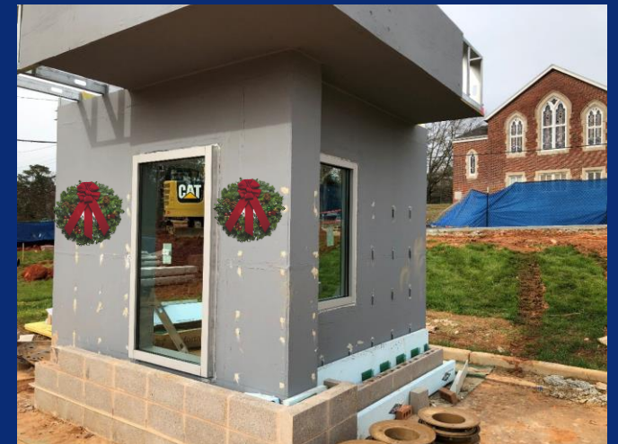
Storefront and curtainwall systems installed on skin mock-up
