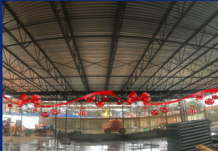
Metal decking installed on lower level
