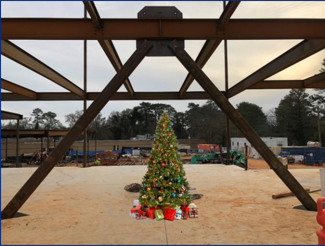
Braced frame on main level west
