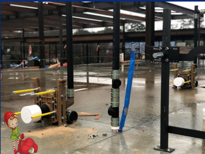
Carriers installed on main level west
