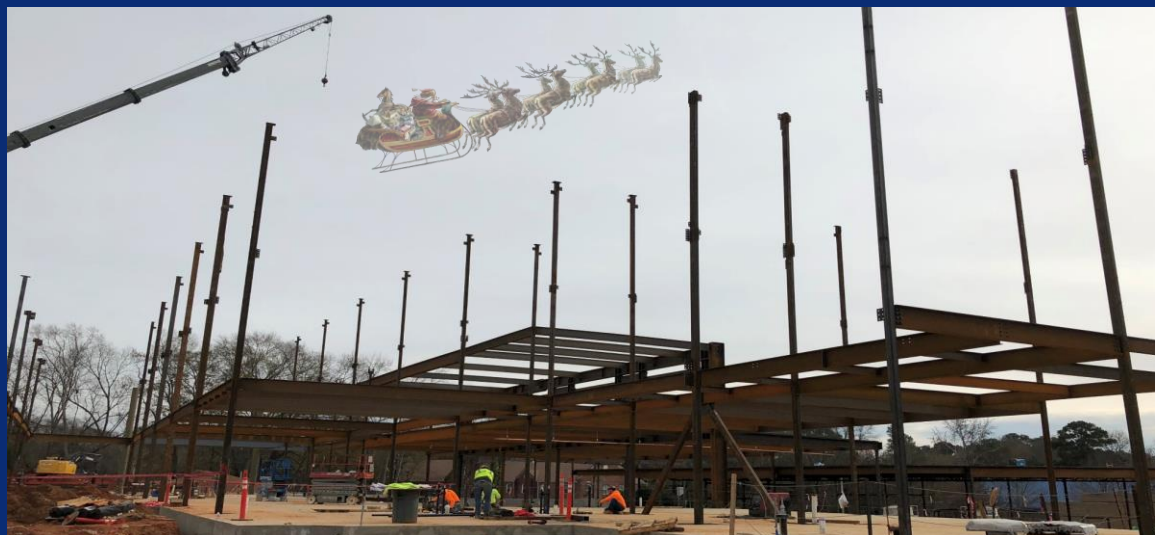
Photo of the project site looking at main level west and sequence 2 steel
