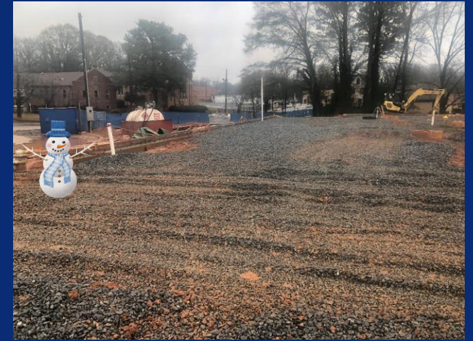
Main level east slab on grade prep
